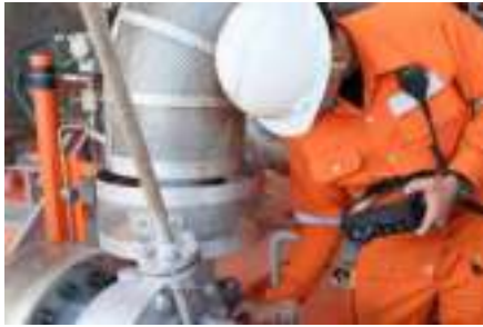
Vibration Troubleshooting & Retrofitting
