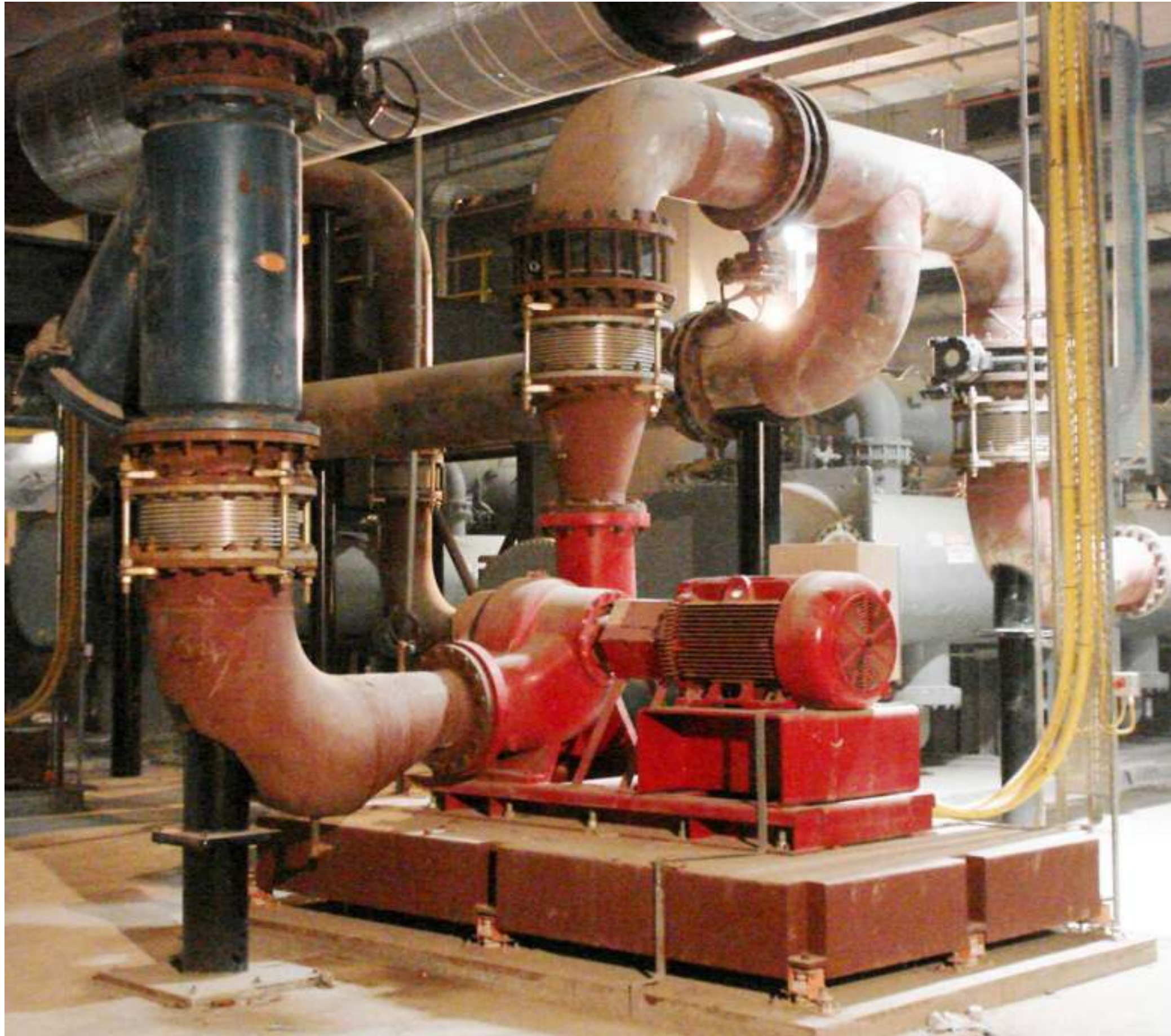
HALOGEN LEAK TESTING
