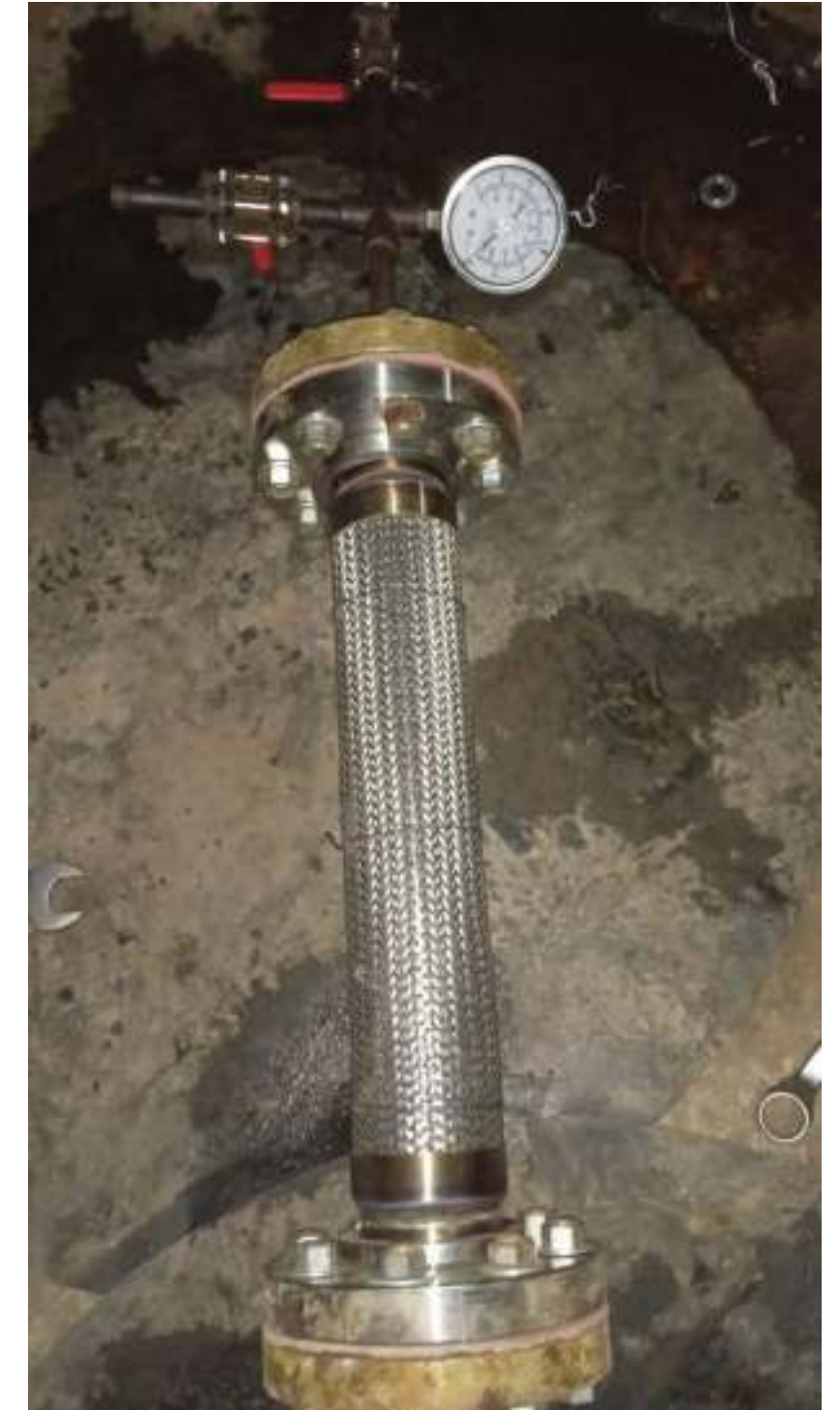
In-house Hydro testing
