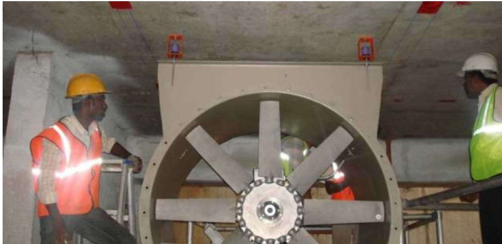
Spring Hangers installed with Axial Fan
