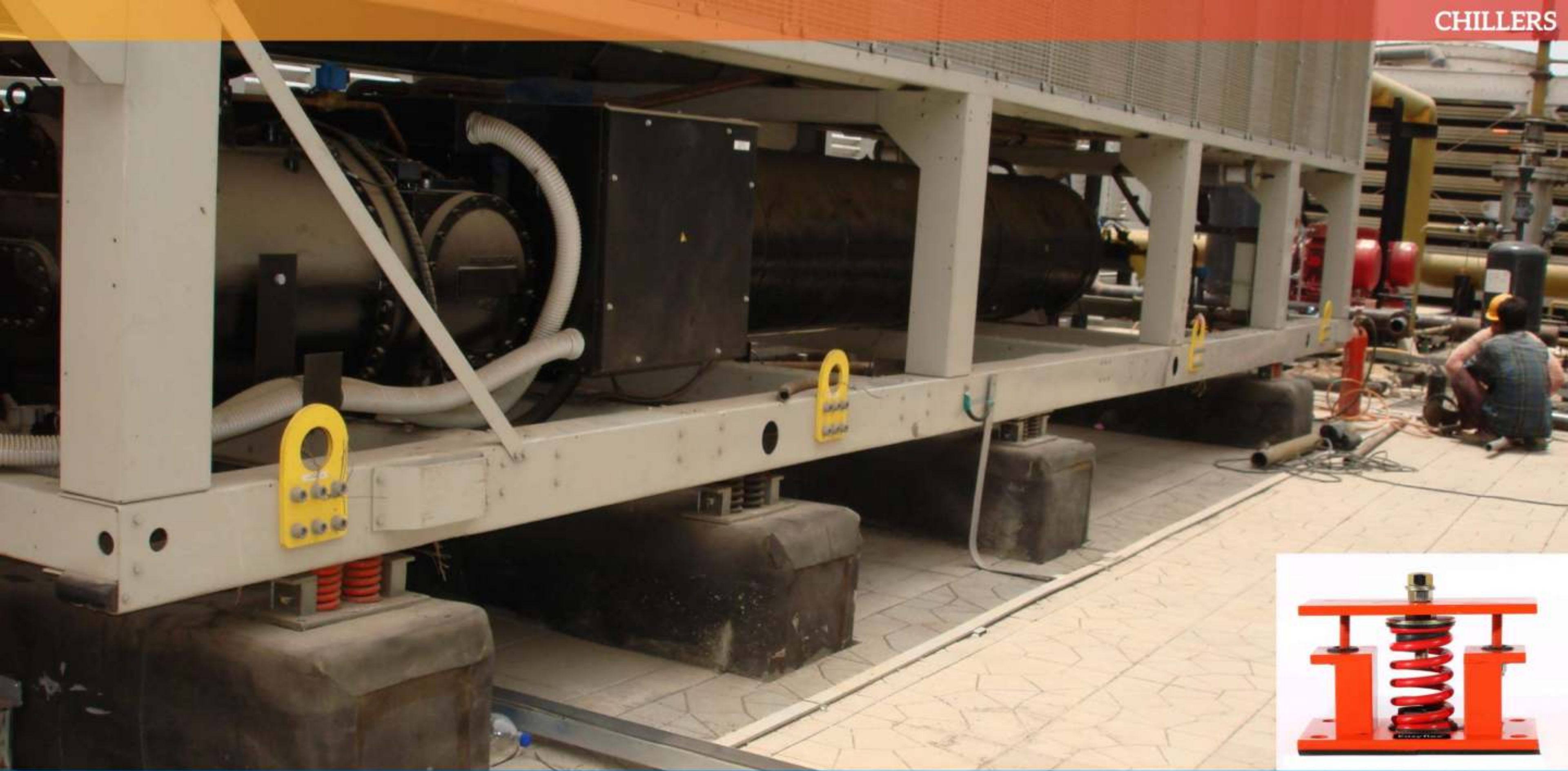
VIBRATION ISOLATION FLOOR MOUNTED | RESTRAINED SPRING ISOLATOR | 9 SPRING MODEL | 10 TON POINT LOAD
