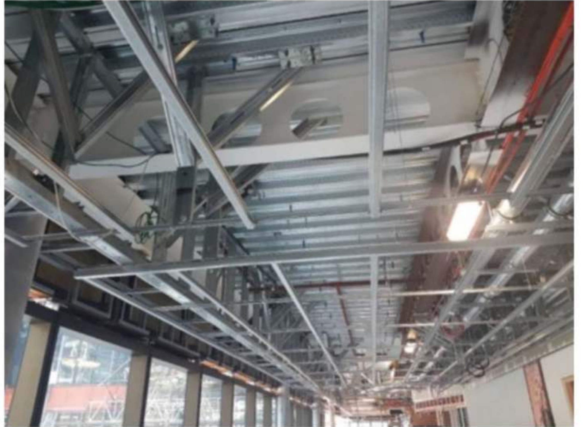
Seismic restraint of Services & Ceiling
