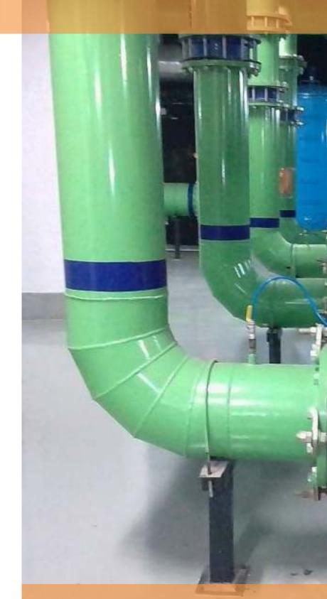
Rubber Expansion Joints installed with CHW Pumps at an International Airport.
